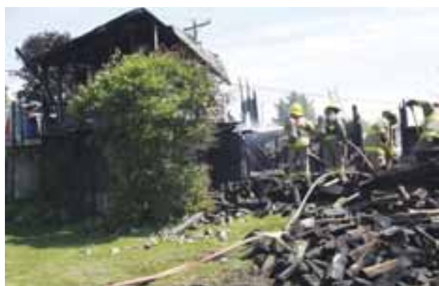
Firefighters extinguish hot spots after a July 4 fire destroyed the home of Gary and Nicole Lamarche on Chemin Pembroke in L'Isle-aux-Allumettes. (PS)
